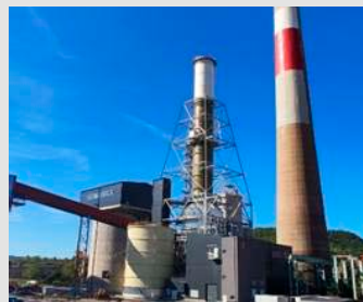
Flue Gas Desulphurization Construction Project for Ugljevik Thermal Power Plant
